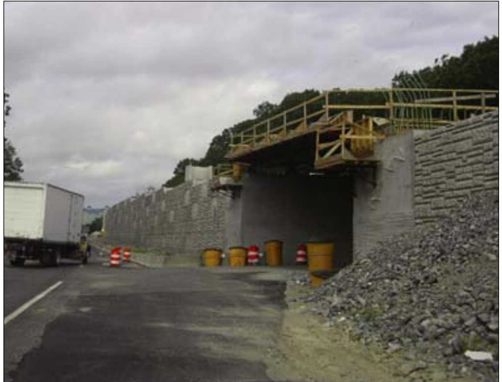
New road construction at Foxwoods Casino
